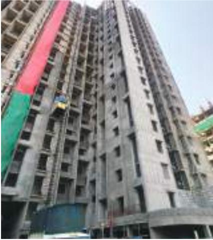
YashONE Wakad Central 'A' - Gypsum plaster work is in progress on 21<sup>st</sup> floor, kitchen otta platform work is in progress on 21<sup>st</sup> floor.
