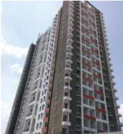
YashONE Hinjawadi 'A' - External painting 2<sup>nd</sup> coat work is in progress, Internal flooring work is in progress on 22<sup>nd</sup> floor, Acid wash has been completed till 7<sup>th</sup>.
