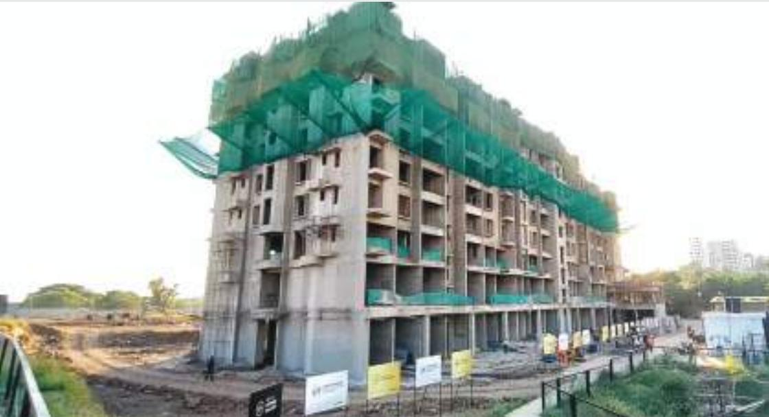
Yashwin Orizzonte 'A' - 8<sup>th</sup> floor slab shuttering work is in progress.
