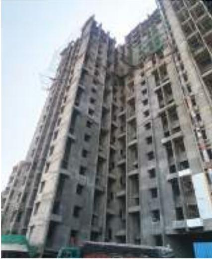
YashONE Wakad Central 'D' - 21<sup>st</sup> floor Slab Pour1 casting has been completed, Pour2 slab shuttering & reinforcement work is in progress, blockwork is in progress on 17<sup>th</sup>.
