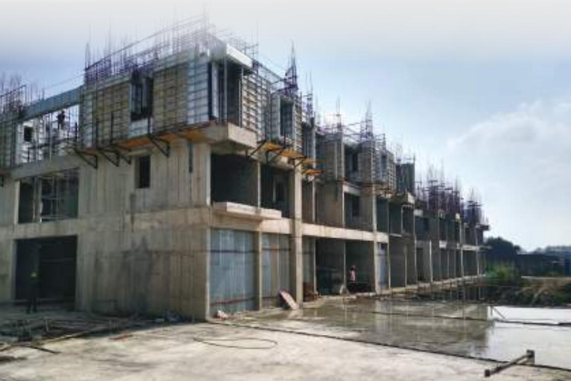
YashONE Infinitee 'C1C2' - 3<sup>rd</sup> floor slab Aluform mockup work is in progress.
