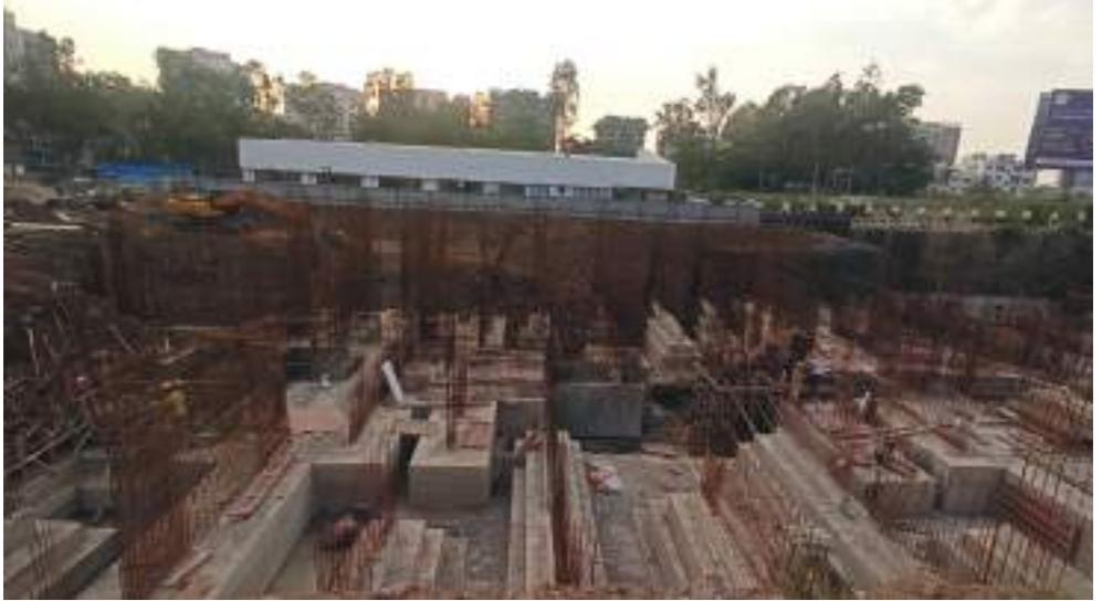
Yashwin Supernova 'C' - Footing casting work has been completed, shearwall reinforcement work is in progress.
