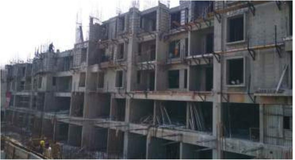
YashONE Infinitee 'D1D2' - 3<sup>rd</sup> floor slab casting work has been completed, 4<sup>th</sup> floor slab shuttering & reinforcement work is in progress.
