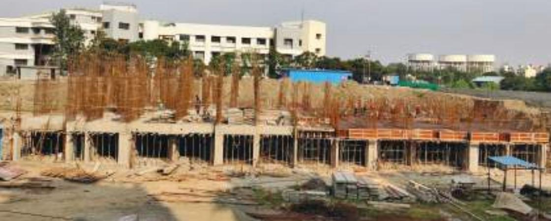
Yashwin Supernova 'A' - Pour 1 - 1<sup>st</sup> slab shearwall reinforcement binding & shuttering work is in progress, Pour 2 - Slab reinforcement & shuttering work is in progress.
