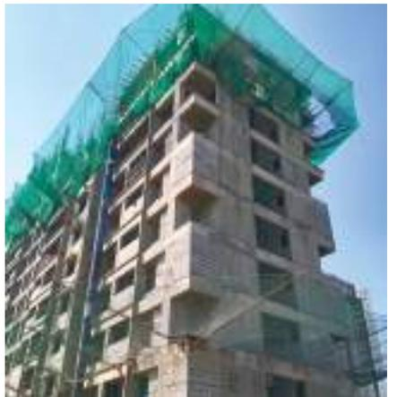
Yashwin Sukhniwas 'D' - 10<sup>th</sup> floor slab casting work is in progress, blockwork is in progress on 6<sup>th</sup> floor, gypsum plaster work is in progress on 5<sup>th</sup> floor.
