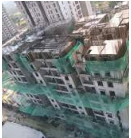
YashONE Hinjawadi 'D' - Part-01 casting work is in progress for 10<sup>th</sup> slab, blockwork is in progress on 2<sup>nd</sup> floor.
