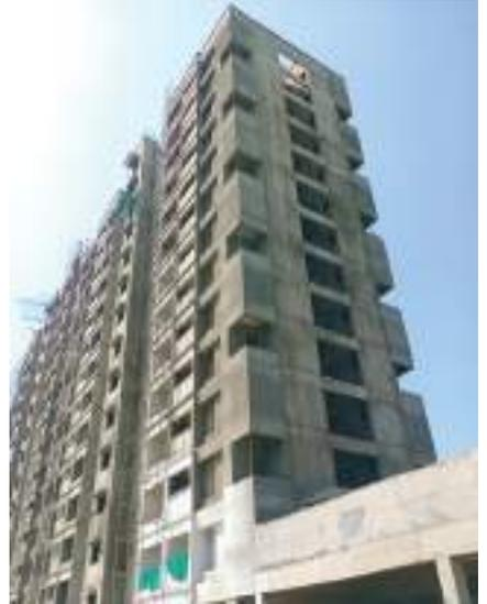
Yashwin Sukhniwas 'B' - OHWT top slab reinforcement work is in progress, blockwork has been completed till 13<sup>th</sup> floor, door frame fixing work is in progress on 4<sup>th</sup>.
